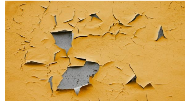
Cracking and peeling (geometry deterioration) of wall paint by weathering
